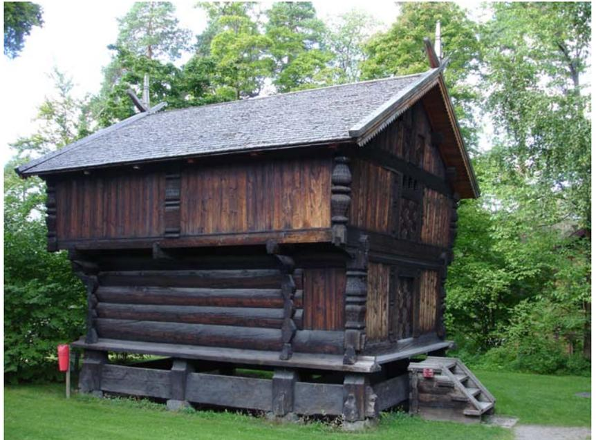
This first picture on the right shows a two storey store-house, made entirely from wood. It dates from the 1700s and was typical of rural buildings, where wood was widely available. The upper level is built with a characteristic overhang. There is an enclosed porch on the front with stairs up to the upper level. Such a store house would have been used to store food for the winter. It is raised above the ground, away from the snow.
