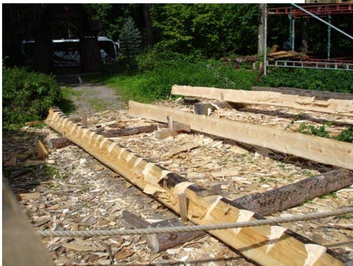
Usually, the wood used for building such as the walls was not seasoned. So allowances had to be made for shrinkage. This could be a problem if vertical timber columns are used in addition to the horizontal members making up the wall, so this needs to be allowed for in the design. (As wood dries, it shrinks more across the grain than lengthways, so the cross pieces can be expected to shrink more the vertical column.)
