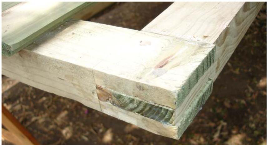
The groove was cut using a Stanley plow plane #??? With a 10mm cutter. There was no power for a router where the screen was assembled, so the groove was cut in-situ, by hand.
