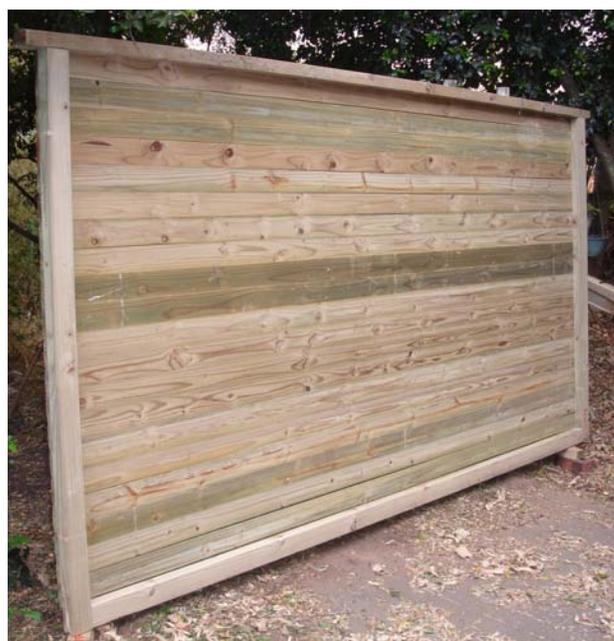
A disadvantage of CCA treated wood, is that it is often delivered with a high moisture content from the treatment process, and as the wood dries, it can warp. CCA treated wood offcuts should be treated as toxic waste – they shouldn't be burned or put onto the compost heap.
