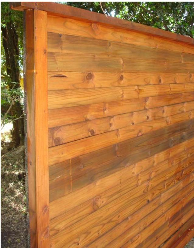
The siding I used has a machined overlap, so the sides locate against each other, to provide some support. I used the straightest pieces to start at the top where they would be most visible and ended up with worst at the bottom. With some judicious clamping, all the pieces fitted together to make a neat siding. The ends of the siding were screwed to the posts using copper-coated decking screws intended for outdoor use.
