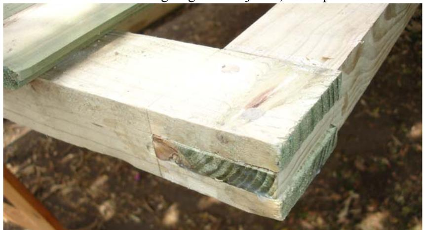
surfaces of both rails were chamfered, so as to shed water.
