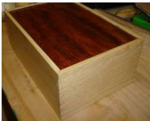
The interior divisions are 5mm pine, dovetailed at the corners and rebated into the sides.
